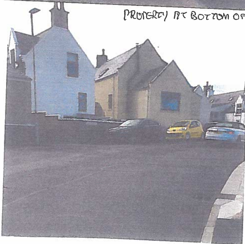
NO 17 HARBOUR PLACE WITH ANTICAPITAL PROPERTY ON Page 52 HARBOUR ROAD WITH GYSEIM UVIC WINDOWS,
