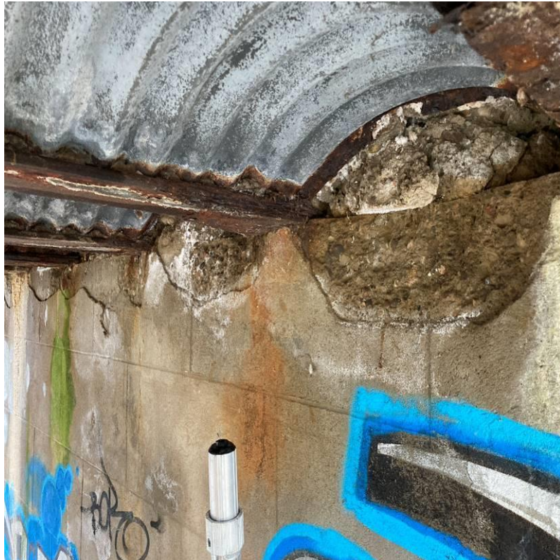
Photograph 40: Significant concrete spalling along top of east abutment between beams in each bay. Aggregate exposed and loose when disturbed.
