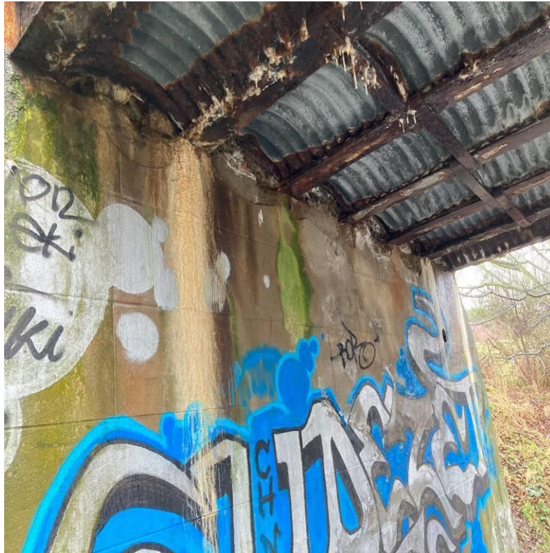
Photograph 39: Significant calcite and algae staining to face of east abutment below support positions of steel beams.
