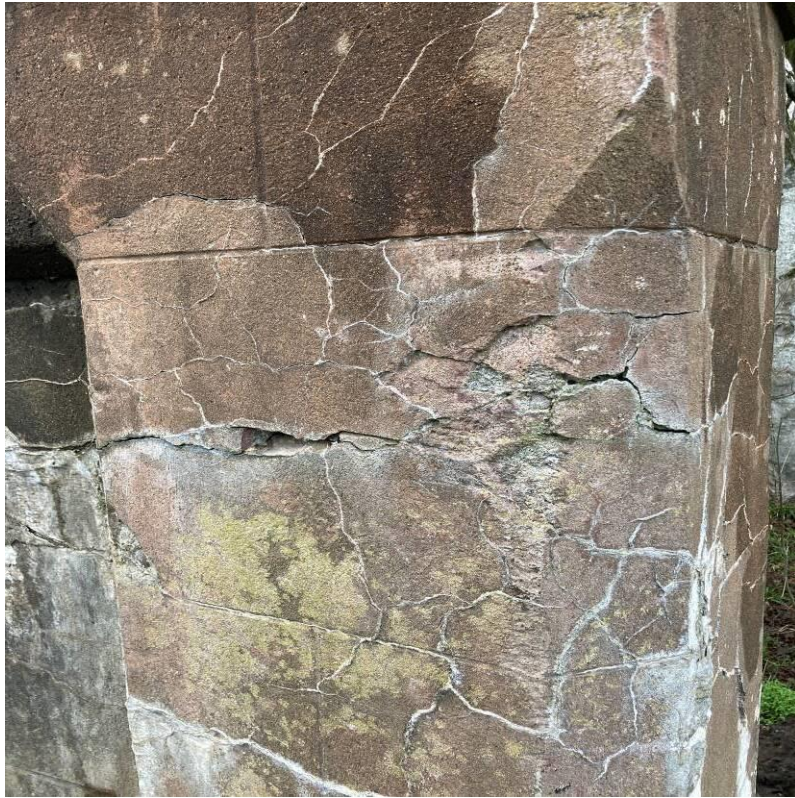
Photograph 25: Evidence of vehicle collision to north-east approach wing wall with spalled concrete and widespread cracking to wall and cope.
