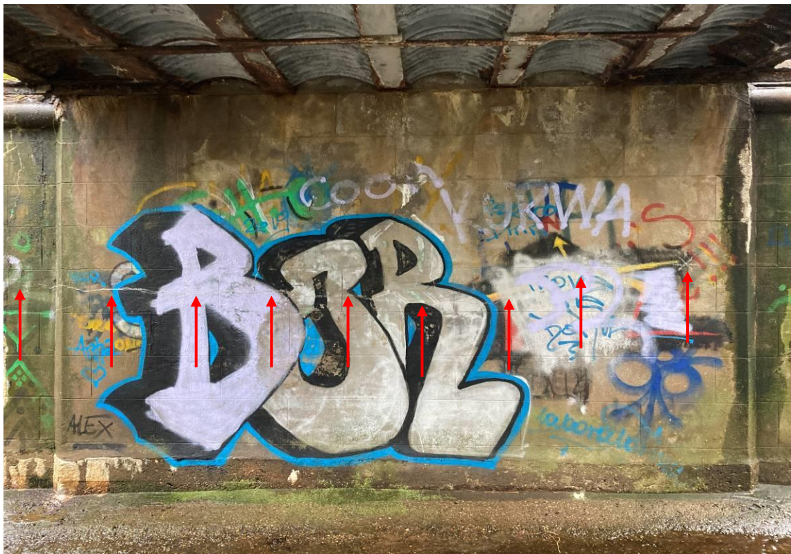
Photograph 46: Horizontal crack propagating full width of western face of Pier 1. Height of crack varies between 1.3m and 1.6m above invert level. Width of crack varies along length but is less than 1mm at all times.
