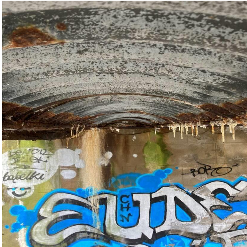
Photograph 7: Widespread calcite stalactites to bottom flange of PB1 – PB7 indicating extensive water ingress through deck structure. Typical localised surface rust at junction between corrugated steel shuttering and steel beam bottom flange.
