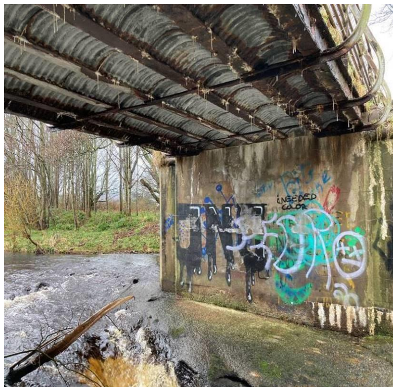
Photograph 8: Widespread calcite stalactites to bottom flange of PB1 – PB7 indicating extensive water ingress through deck structure.
