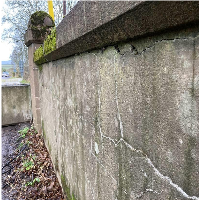
Photograph 23: Typical widespread hairline cracking to approach wing walls.
