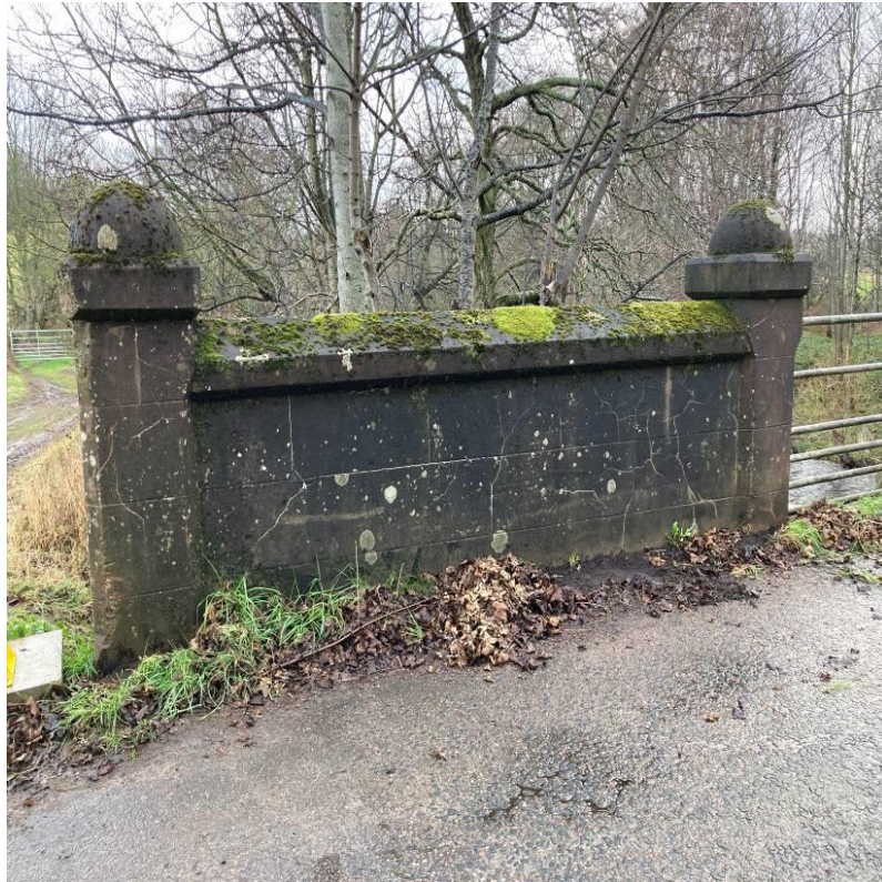
Photograph 22: Typical widespread hairline cracking to approach wing walls.
