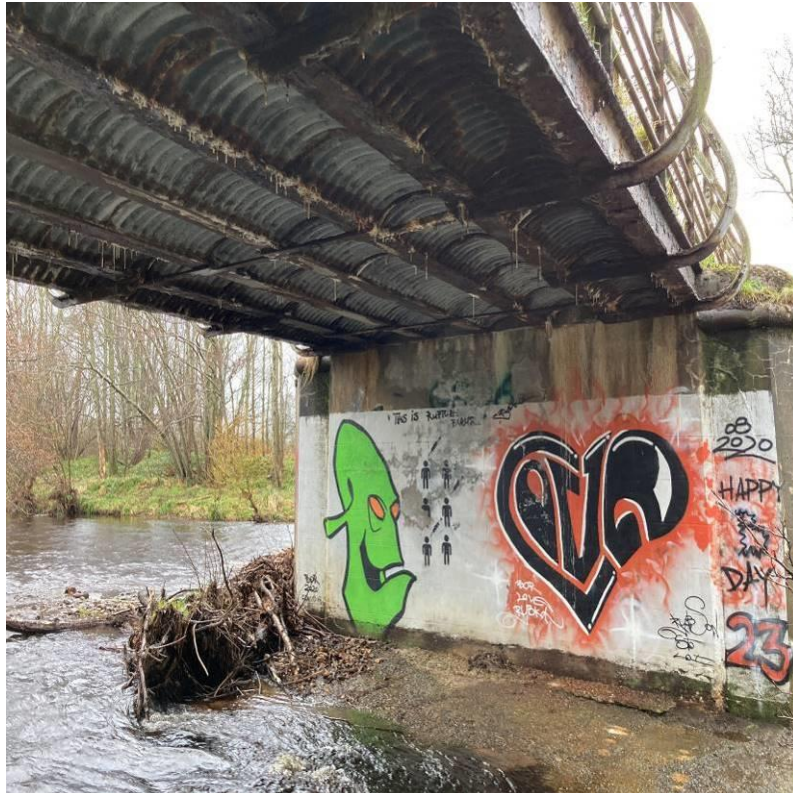
Photograph 34: Accumulation of vegetation to upstream cutwater of Pier 2.
