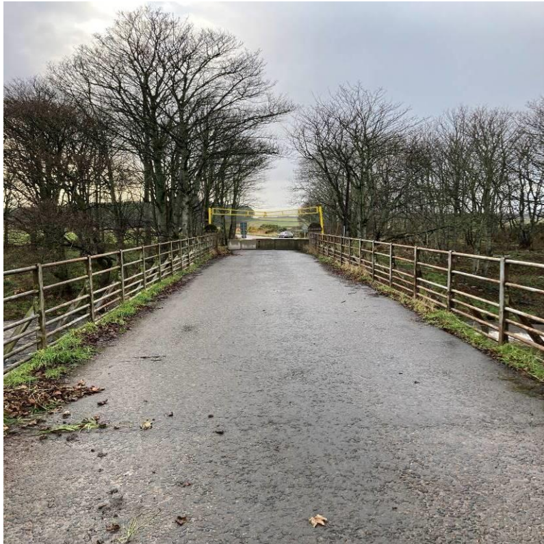
Photograph 26: Typical band of vegetation growth within drainage channel to carriageway edge.
