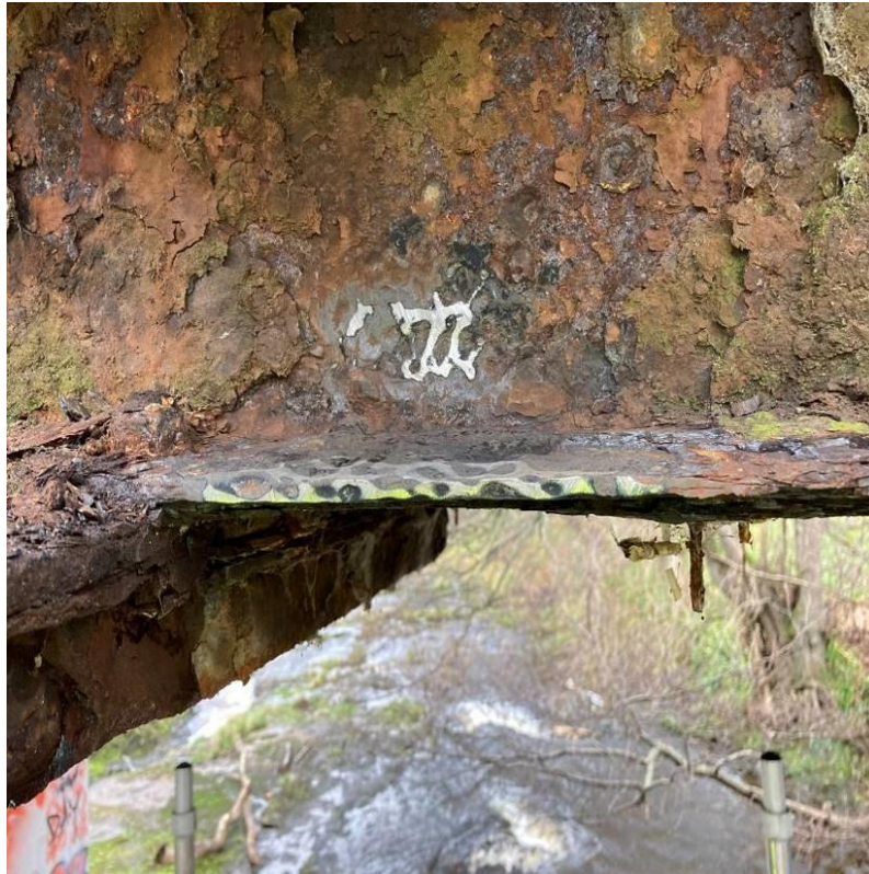
Photograph 5: Visible section loss to flange of PB1 & PB7 over all three spans. Flange measuring 4-6mm at toe and, on average, 12.4mm at quarter points of overall flange width.
