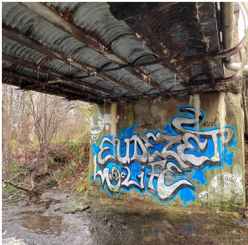
Photograph 38: Significant calcite and algae staining to face of east abutment below support positions of steel beams.
