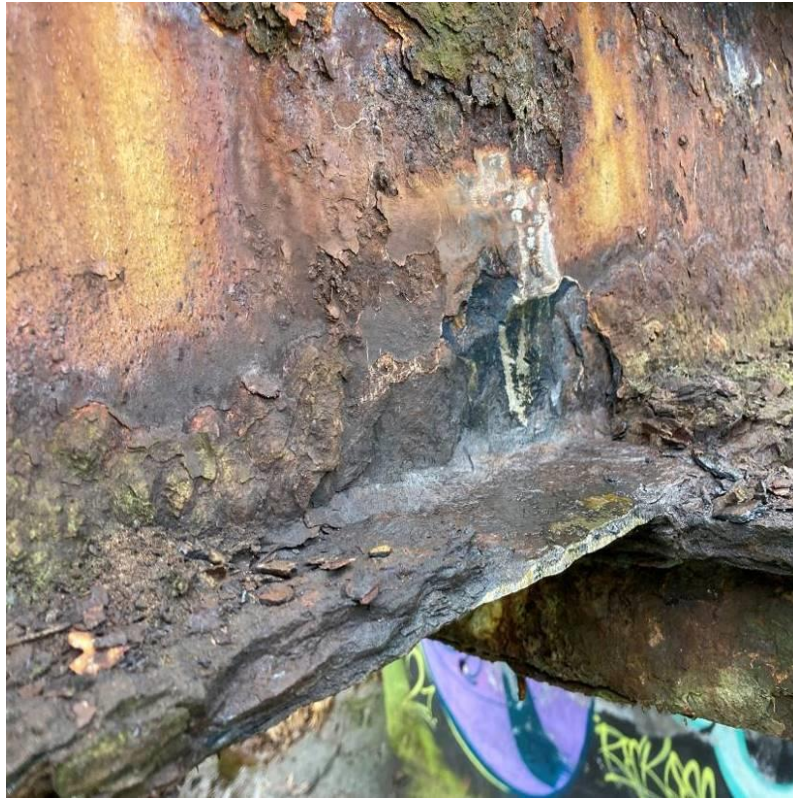
Photograph 3: Widespread corrosion, delamination and layered rust build up to entire length of exposed web and flange of PB1 & PB7 over all three spans.
