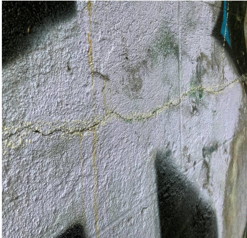
Photograph 47: Horizontal crack propagating full width of western face of Pier 1. Height of crack varies between 1.3m and 1.6m above invert level. Width of crack varies along length but is less than 1mm at all times.
