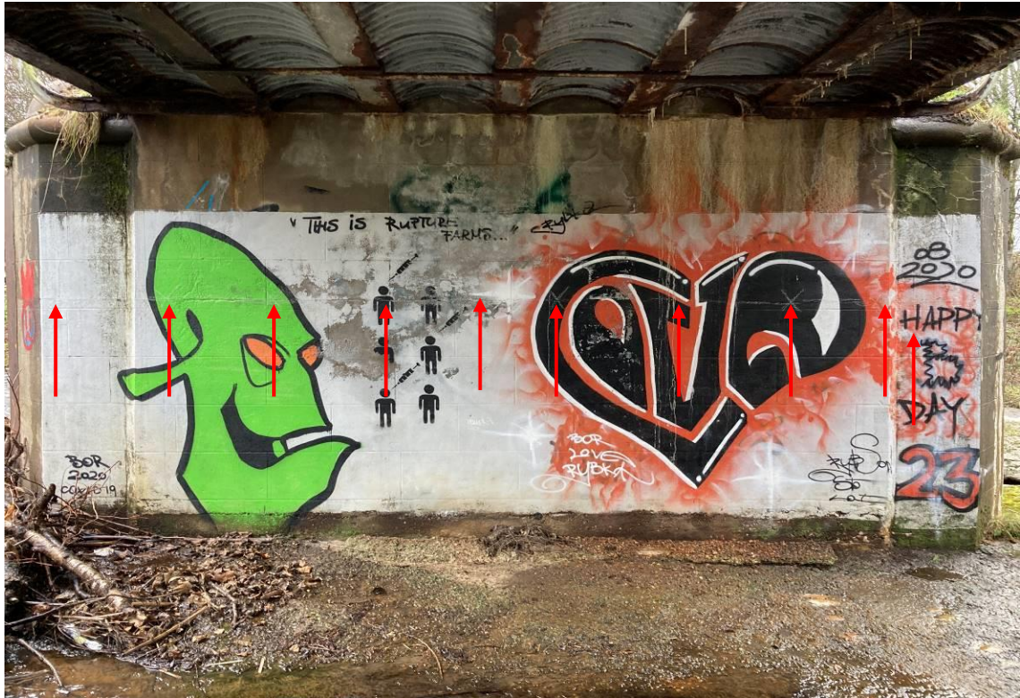
Photograph 51: Horizontal crack propagating full width of eastern face of Pier 2. Height of crack varies between 1.3m and 1.6m above invert level. Width of crack varies along length but is less than 1mm at all times. Typical calcite staining to face of Pier 1 and Pier 2.
