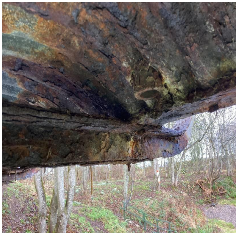
Photograph 30: Widespread corrosion, delamination and layered rust build-up to lower section of parapet brace member.
