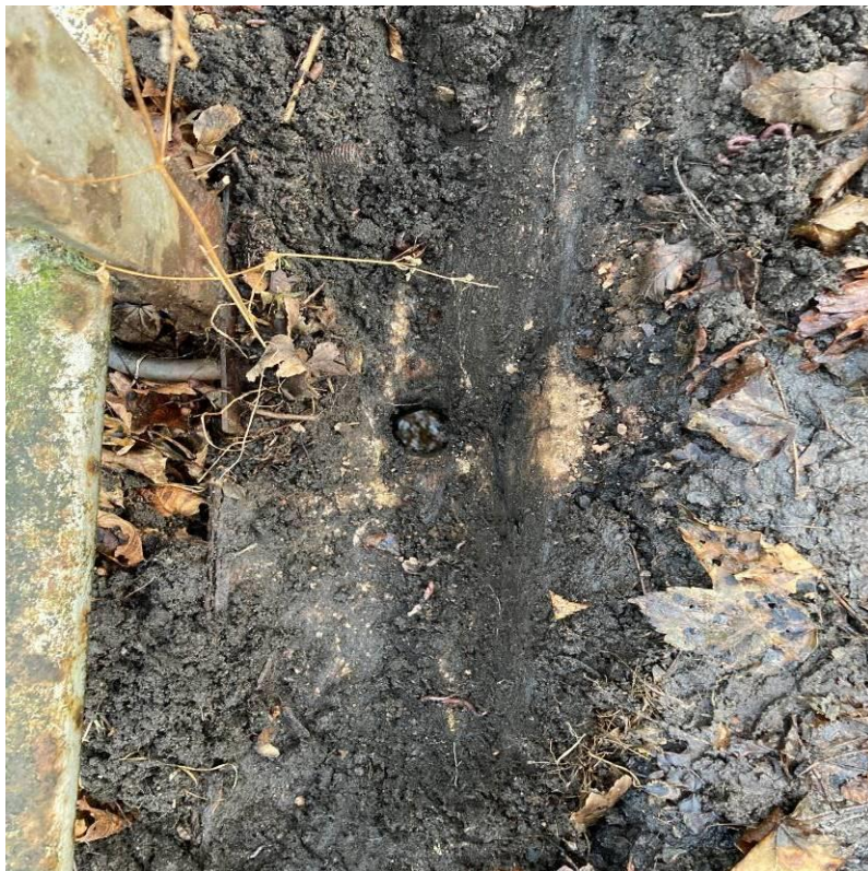
Photograph 28: Typical drainage outlet situated to north and south of bridge at mid-point of each span. Typically blocked by silt and vegetation.
