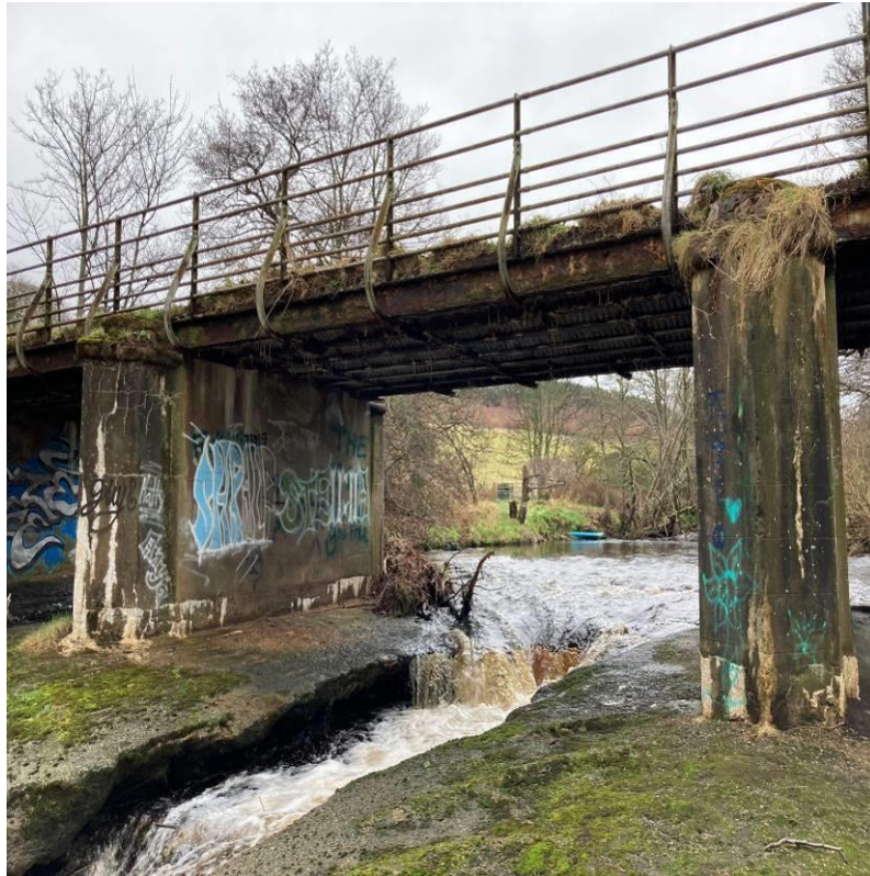
Photograph 33: Visible cut in concrete invert below Span 2 with fast flowing water. Extent of scour below invert unclear. Accumulation of vegetation to upstream cutwater of Pier 2.
