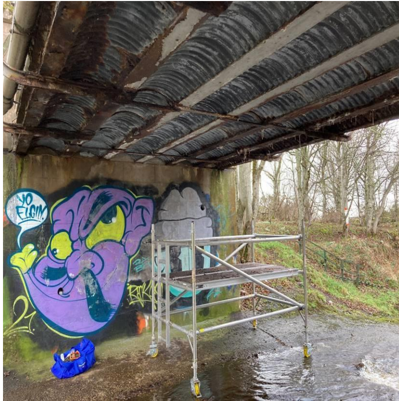
Photograph 37: Damp and algae staining to face of west abutment below support position of PB1 and PB7. Two 100mm diameter cores noted to face of abutment extending 700mm back into structure.
