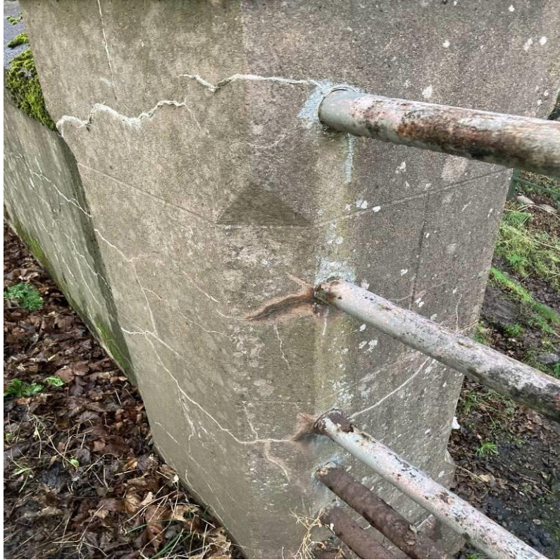
Photograph 21: Typical cracks propagating from the junction between the steel parapet rails and mass concrete approach wing walls.
