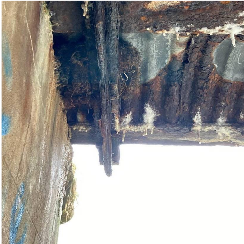
Photograph 32: Vegetation due to nesting birds resting on parapet brace to east and west of Span 2.
