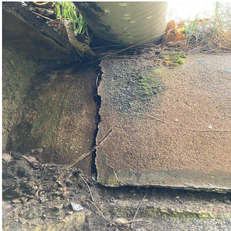
Photograph 52: Typical concrete breakout and cracking with vegetation growth to decorative cutwater capping.
