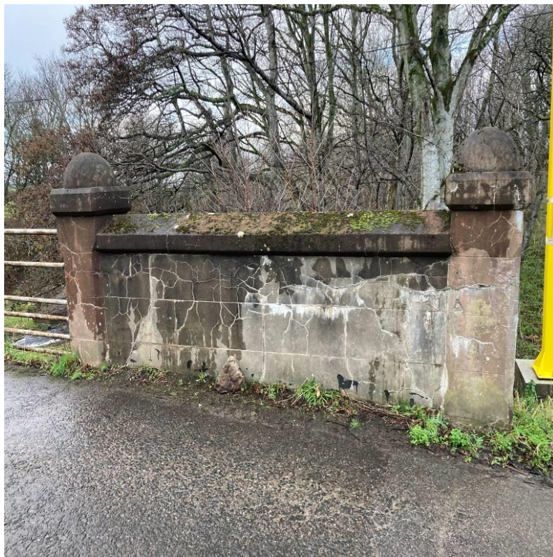
Photograph 24: Evidence of vehicle collision to north-east approach wing wall with spalled concrete and widespread cracking to wall and cope.
