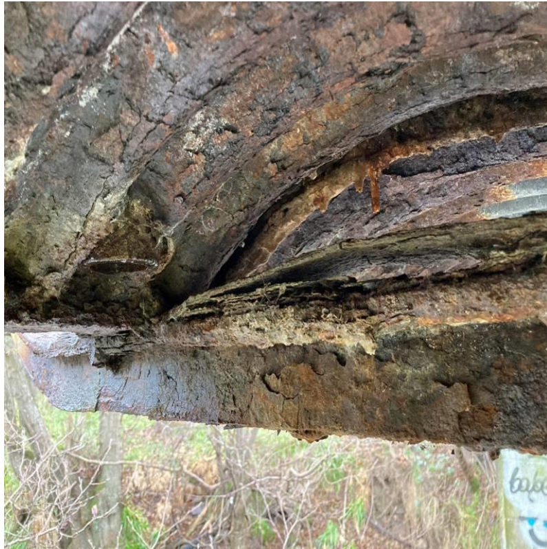
Photograph 31: Widespread corrosion, delamination and layered rust build-up to lower section of parapet brace member.
