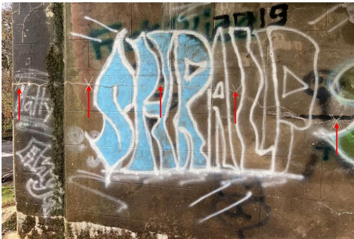
Photograph 50: Horizontal crack propagating full width of western face of Pier 2. Height of crack varies between 1.3m and 1.6m above invert level. Width of crack varies along length but is less than 1mm at all times.
