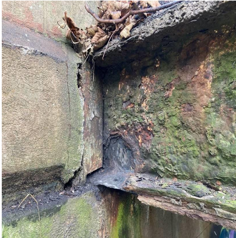
Photograph 1: Widespread corrosion, delamination and layered rust build-up to entire length of exposed web and flange of PB1 & PB7 over all three spans.
