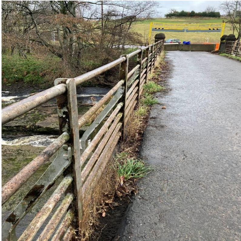
Photograph 19: Typical weathering, surface rust and failure of coating system to parapet rails and upstands.
