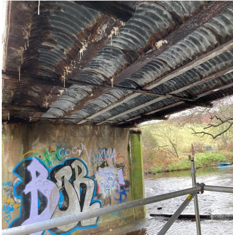
Photograph 11: Flaking paint to soffit of bottom flange of PB4-PB6 in Span 1. Indicative of condition where paint coating was partially intact throughout all three spans.
