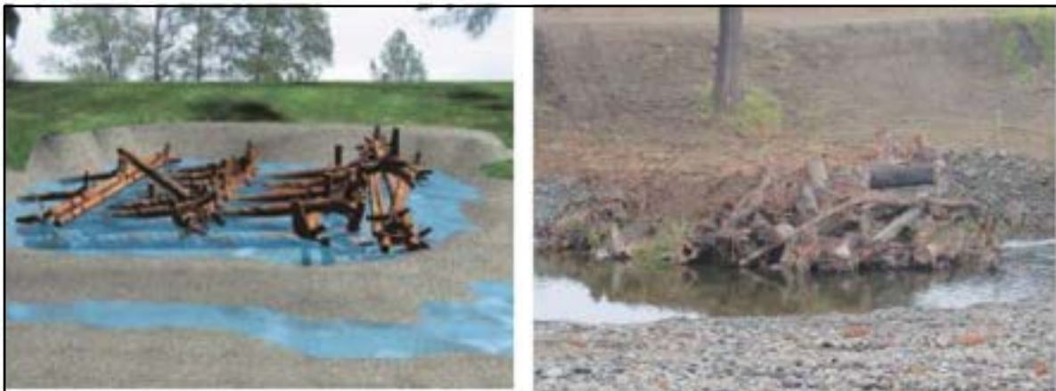
Figure 6.1: Examples of engineered log jam flow deflectors (from Brooks, A. P. 2006)
