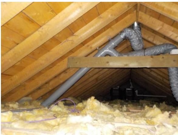
Internal view of roof structure.
