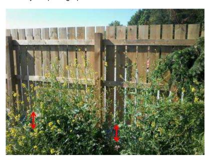
Plate 1: Gap at bottom of fencing as a result of the removal of the lower section
