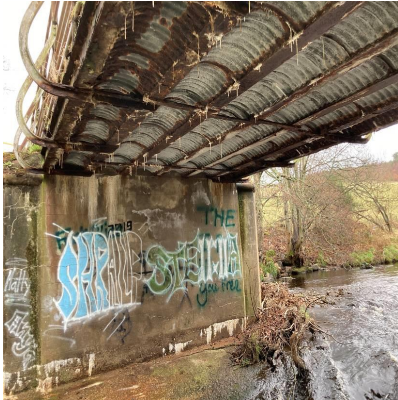
Photograph 13: Surface rust, delamination and corrosion to the corrugated steel shuttering forming the soffit of the structure. Predominant in arches between PB1 - PB2 and PB6 - PB7.
