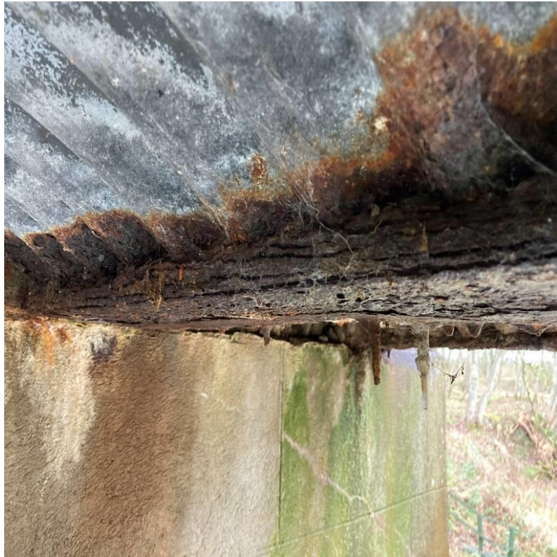
Photograph 14: Typical localised surface rust at junction between corrugated steel shuttering and steel beam bottom flange.
