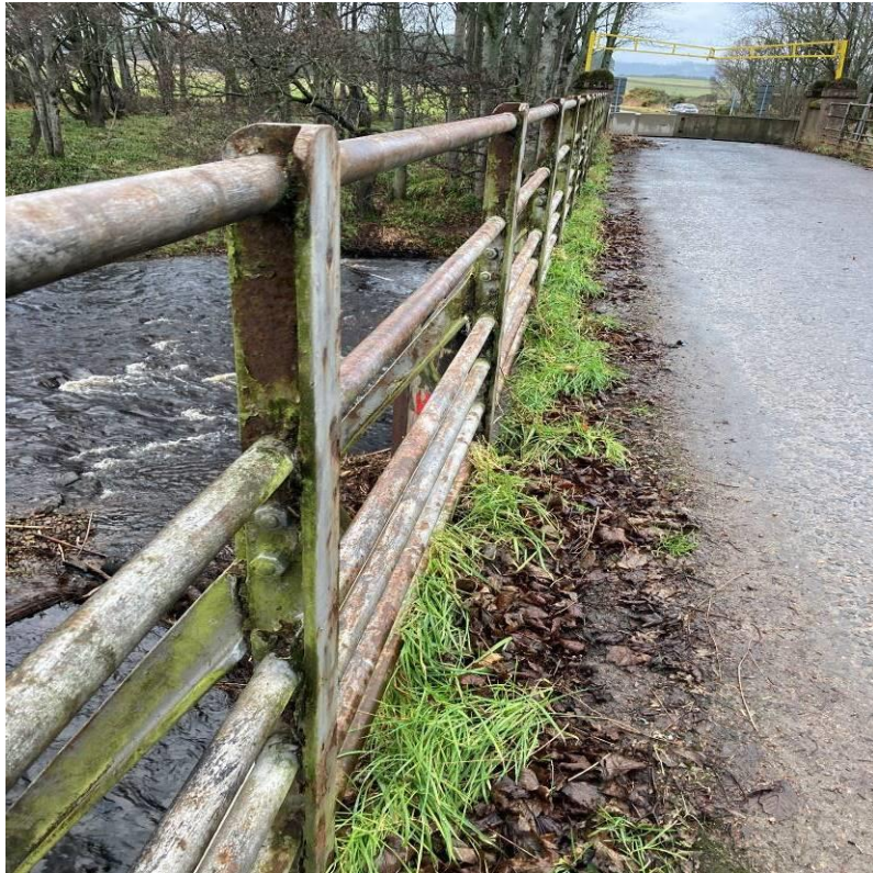
Photograph 20: Typical weathering, surface rust and failure of coating system to parapet rails and upstands.
