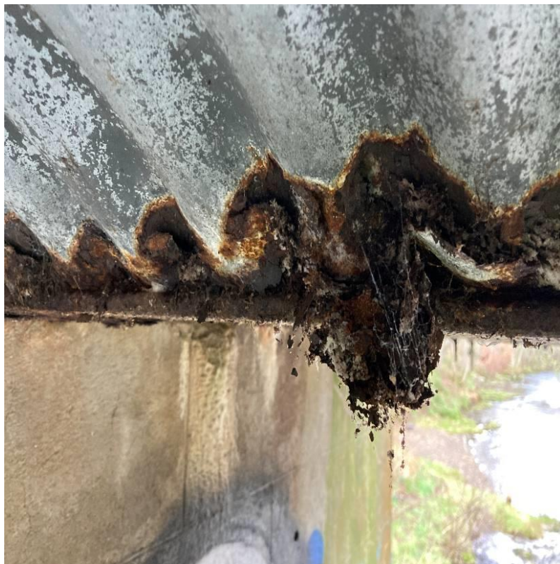
Photograph 16: Localised failure of corrugated steel shuttering at junction with PB3 within Span 1.
