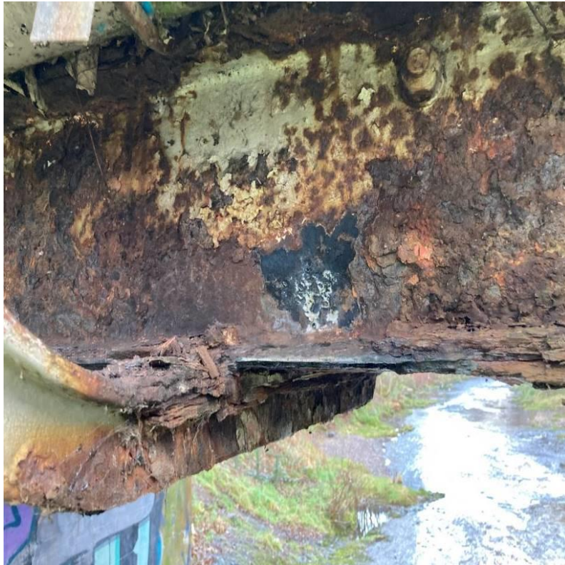
Photograph 2: Widespread corrosion, delamination and layered rust build up to entire length of exposed web and flange of PB1 & PB7 over all three spans.
