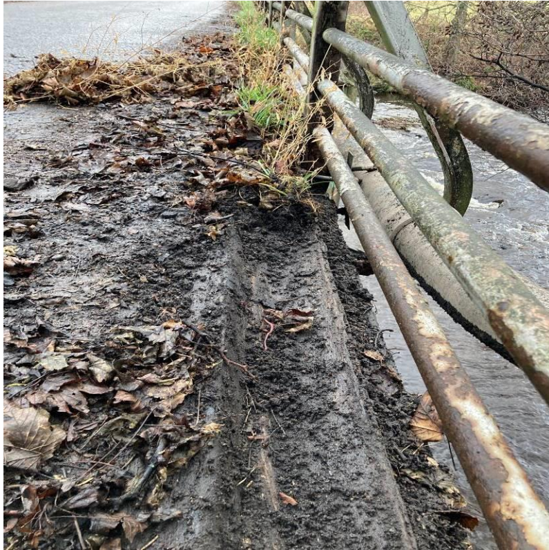
Photograph 27: Typical band of vegetation growth within drainage channel to carriageway edge.
