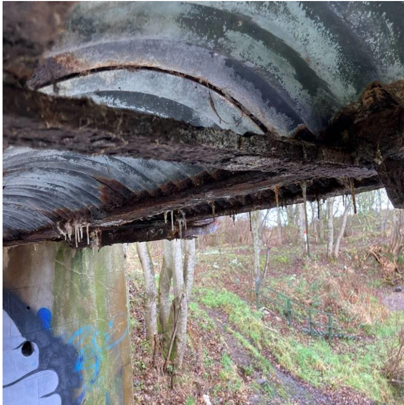
Photograph 4: Widespread corrosion, delamination and layered rust build up to entire length of visible bottom flange of PB2 & PB6 over all three spans.
