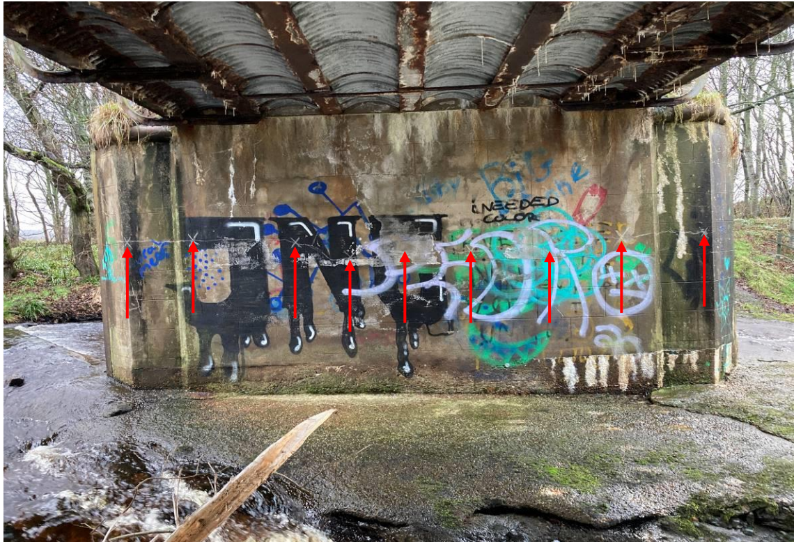
Photograph 48: Horizontal crack propagating full width of eastern face of Pier 1. Height of crack varies between 1.3m and 1.6m above invert level. Width of crack varies along length but is less than 1mm at all times. Typical calcite staining to face of Pier 1 and Pier 2.
