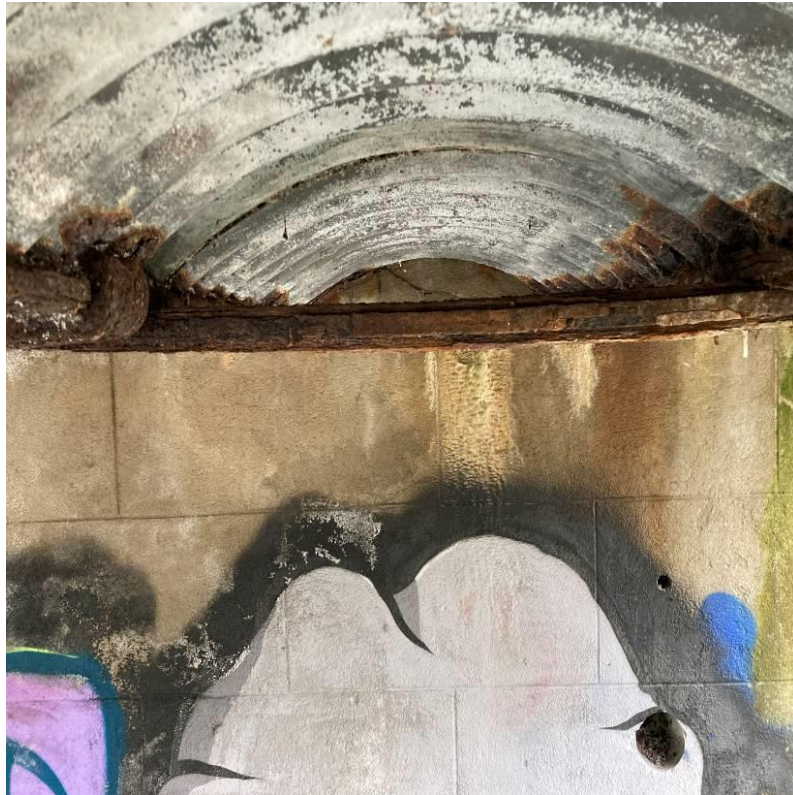
Photograph 18: Typical layered surface rust and delamination to all transverse ties.
