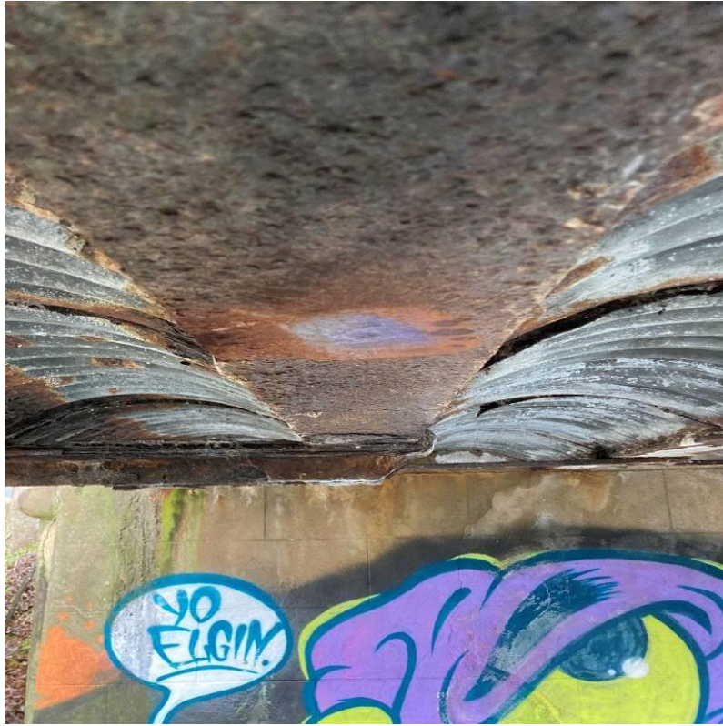
Photograph 9: Typical defect to internal beams - moderate surface rust and pitting to soffit of bottom flange (PB6, Span 1 shown).
