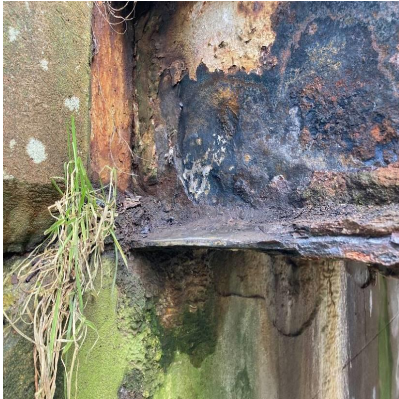
Photograph 6: Widespread corrosion, delamination and layered rust build up to entire length of exposed web and flange of PB1 & PB7 over all three spans.
