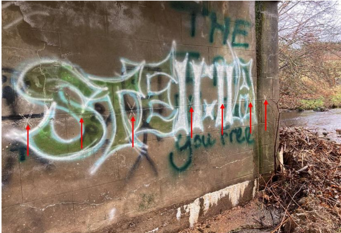
Photograph 49: Horizontal crack propagating full width of western face of Pier 2. Height of crack varies between 1.3m and 1.6m above invert level. Width of crack varies along length but is less than 1mm at all times.
