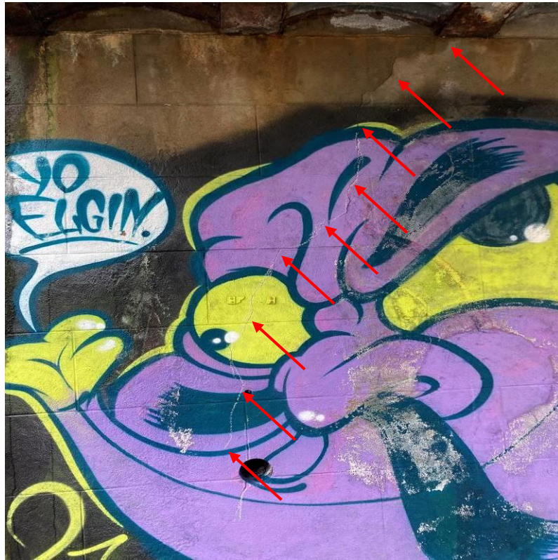
Photograph 35: Vertical crack emanating from the support position of PB5 to approximately 950mm above invert level to west abutment. Crack width measured to be approximately 1mm. Historic crack monitor in state of disrepair.
