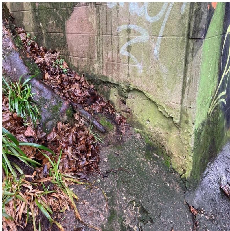
Photograph 36: Typical scour to render at base of west abutment.
