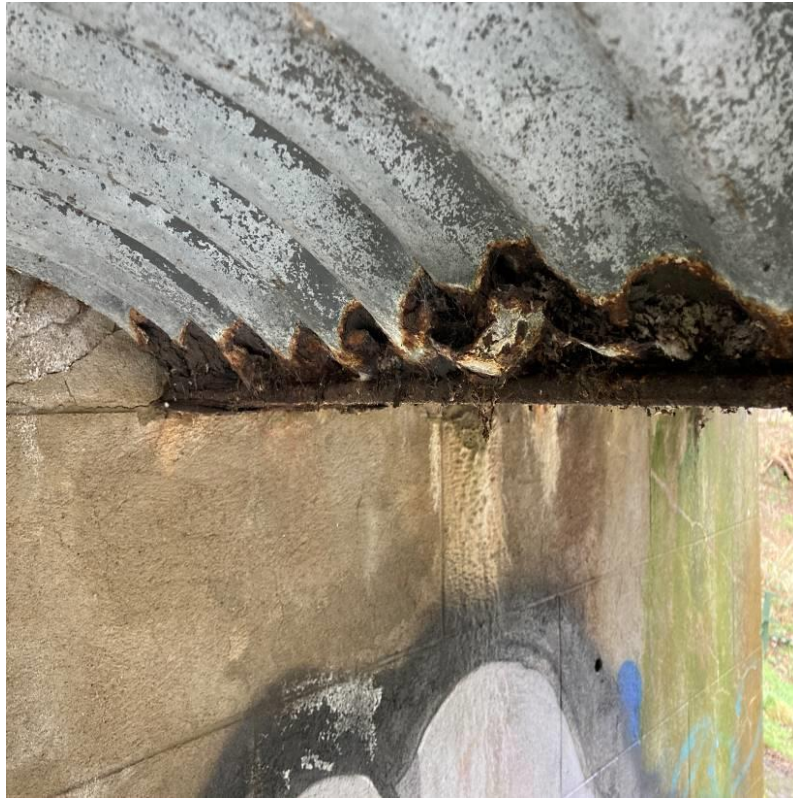
Photograph 15: Localised failure of corrugated steel shuttering at junction with PB3 within Span 1.
