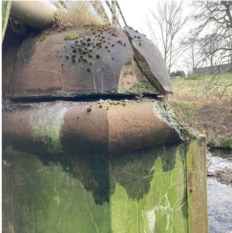
Photograph 53: Typical concrete breakout and cracking with vegetation growth to decorative cutwater capping.
