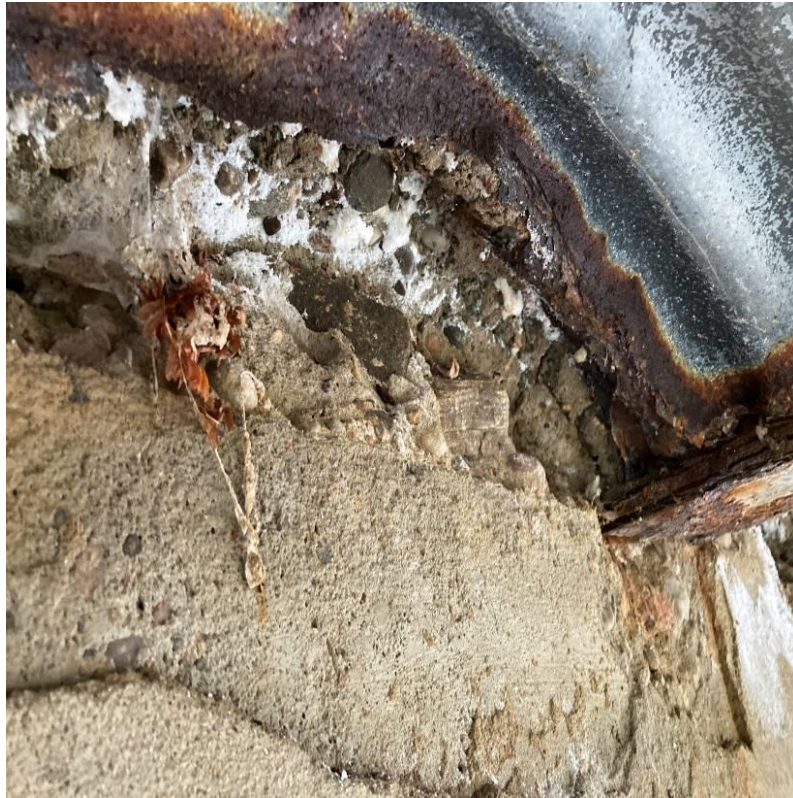
Photograph 17: Mass concrete jack arched slab visible with rounding river gravel aggregate indicating a low grade concrete mix.
