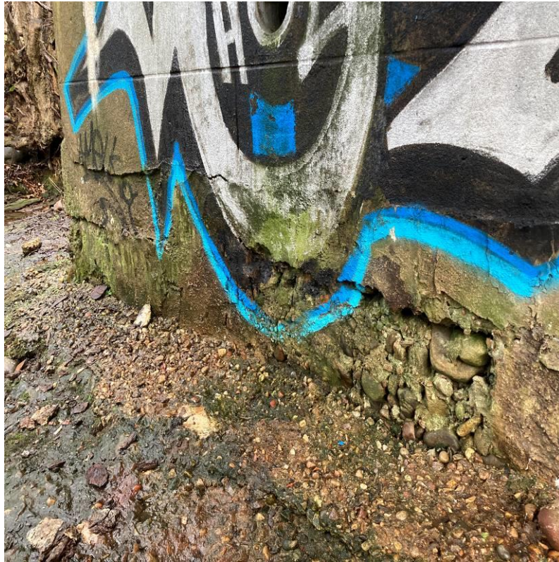
Photograph 43: Typical scour to base at base of east abutment with exposed aggregate.
