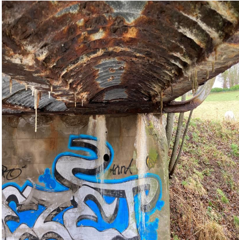
Photograph 12: Surface rust, delamination and corrosion to the corrugated steel shuttering forming the soffit of the structure. Predominant in arches between PB1 - PB2 and PB6 - PB7.
