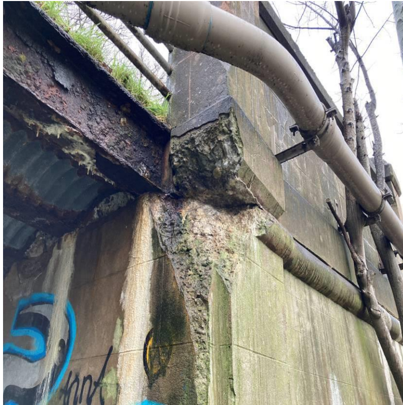
Photograph 41: Significant concrete spalling to south-east corner of east abutment leaving approach wing wall partially unsupported.
