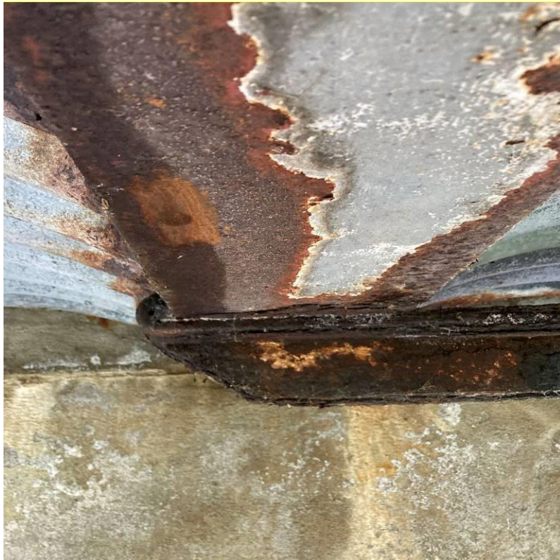
Photograph 10: Flaking paint to soffit of bottom flange of PB4-PB6 in Span 1. Indicative of condition where paint coating was partially intact throughout all three spans.
