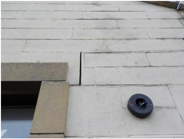
Open joints northeast side.
