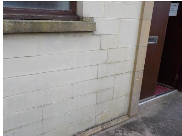
Joint cracking east gable.
