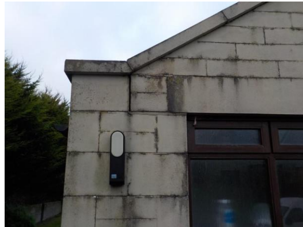
Open joints southeast side.
