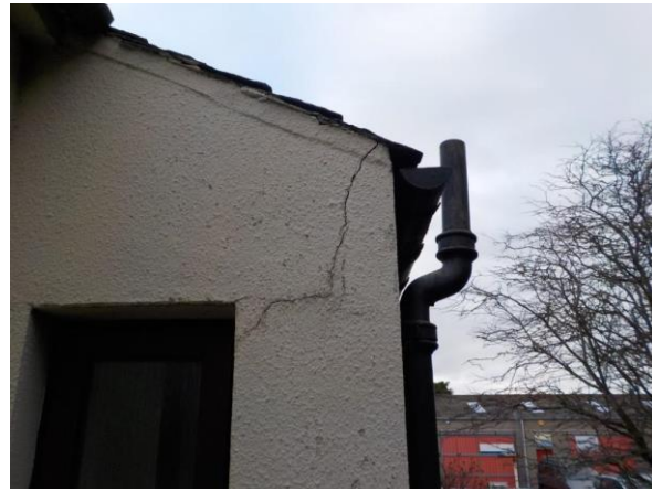
Cracking of side extension east end.
