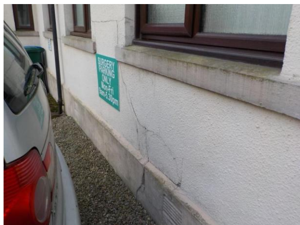
Cracking to west end.
