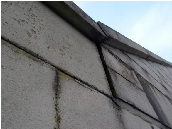
Lateral movement southeast side.
