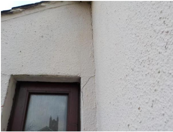
Cracking of side extension east end.
