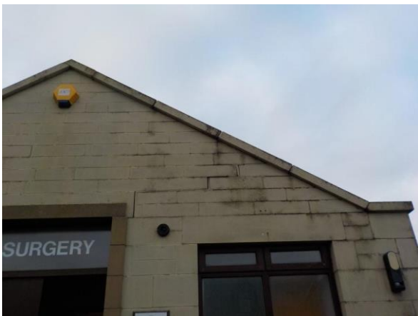
Open joints northeast side.
