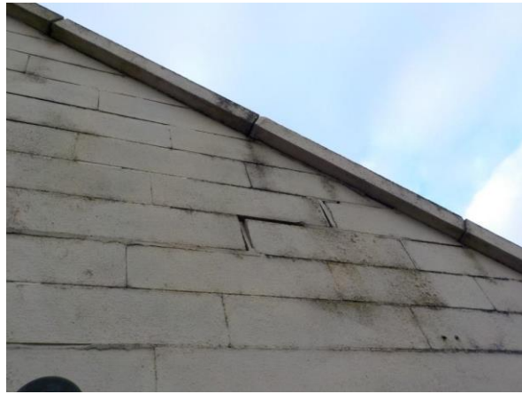
Open joints northeast side.
