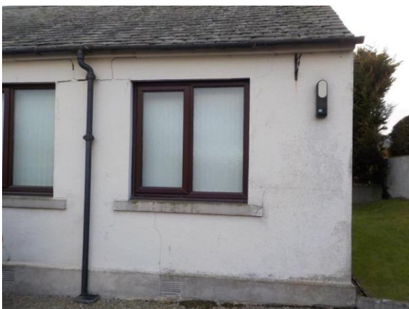
Cracking to west end.
