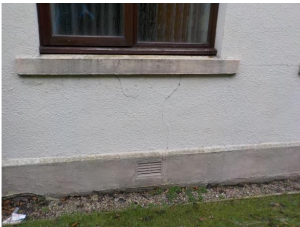
Cracking to south elevation.
