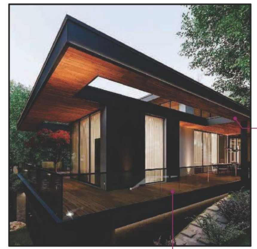
Cedar linings to underside of soffit
