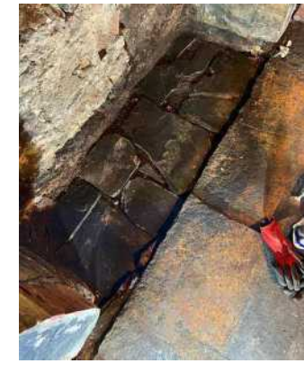
040 east living room original slate hearth bed exposed during 2022 part made up of roofing slates
