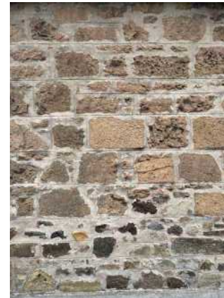
009 front north elevation cherry-cocking stone detail
