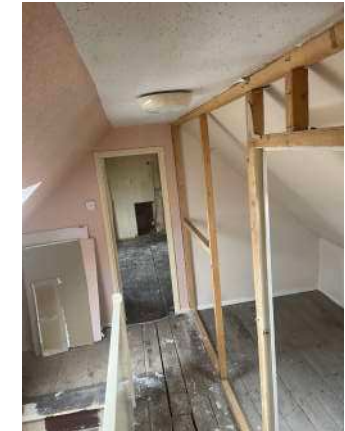
061 first floor landing/passage/stair removing partition wall 2021
