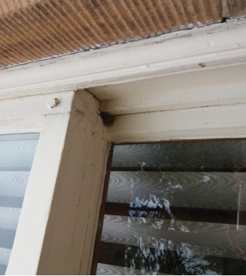
South Elevation bay window, window frames bolted together, joints springing.
