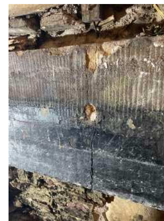
076 cracked fireplace lintel to east living room fireplace
