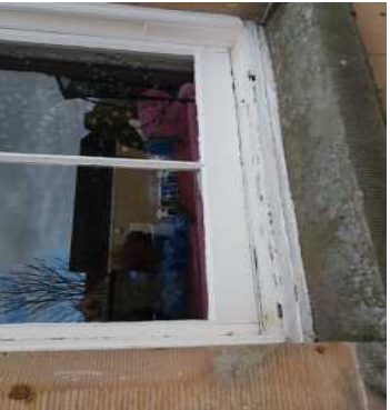
North Elevation bay window, rotten cill ,window frame, sash boxes
