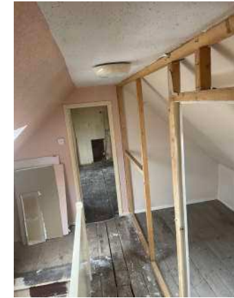
061 first floor landing/passage/stair removing partition wall 2021
