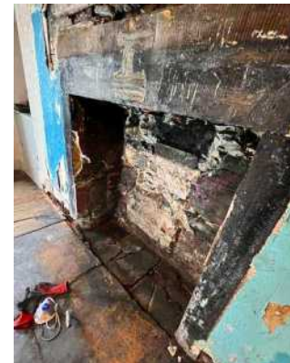
039 east living room fireplace repairs during 2021
