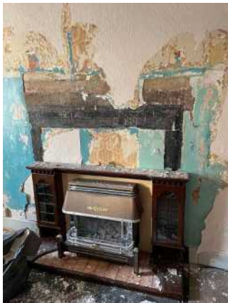
036 east living room original gas fire back boiler during removal 2021
