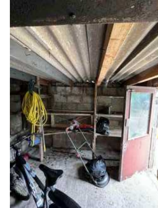
029 north elevation inside garden store
