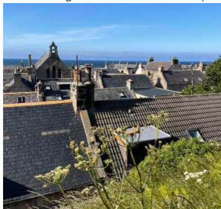
Portgordon varied roofscape
