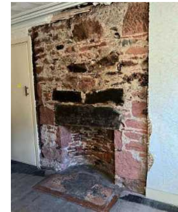
045 west living room fireplace reopened
