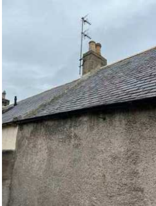
021 south elevation - west chimney
