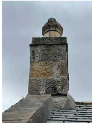
012 east gable chimney
