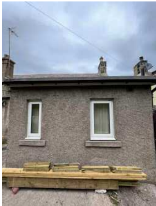
016 south elevation bathroom
