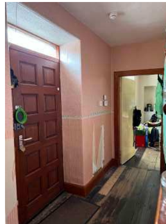
056 entrance lobby view east
