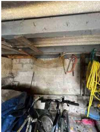
026 west elevation inside garden store
