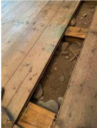
066 void under kitchen floor
