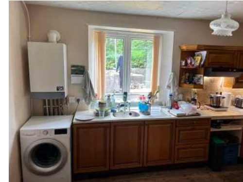
053 kitchen view south
