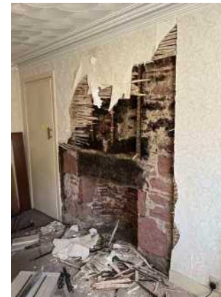
044 west living room fireplace opening removing stone fill during 2022
