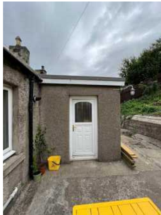
017 west elevation bathroom
