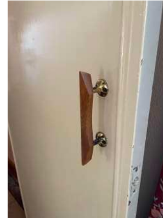
069 ground floor internal door pull handles
