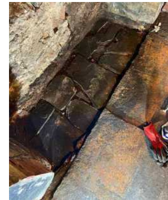
040 east living room original slate hearth bed exposed during 2022 part made up of roofing slates
