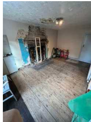
038 east living room fireplace repairs during 2021
