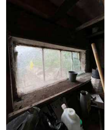
025 east garden store window inside - steel
