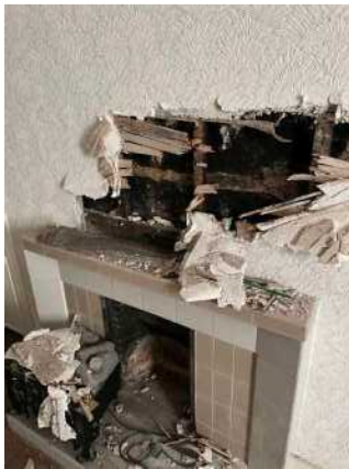
041 west living room fireplace repairs during 2021
