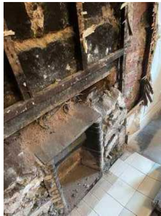
042 west living room fireplace opening removing 1930-50s surround during 2022
