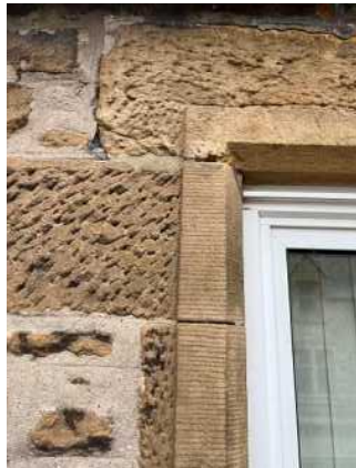
007 front window jamb/lintel stone detail
