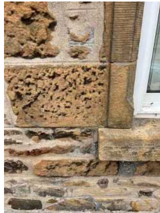
008 front window jamb/lintel stone detail
