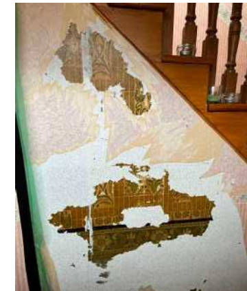
050 front north entrance lobby view south stair wall wallpaper layers
