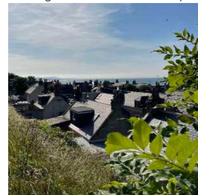
Portgordon varied roofscape
