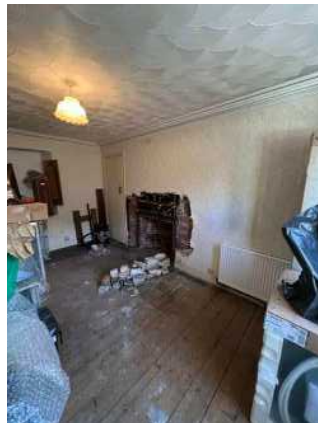
047 west living room fireplace opening removing stone fill during 2022
