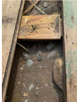
067 void under kitchen floor
