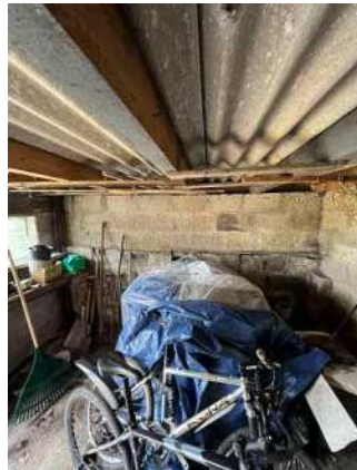
027 south elevation inside garden store
