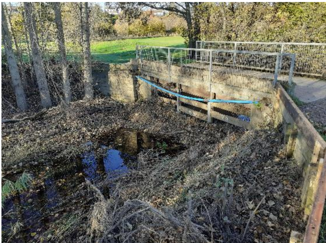
Photo 6 Showing blocked Trash Screen.
