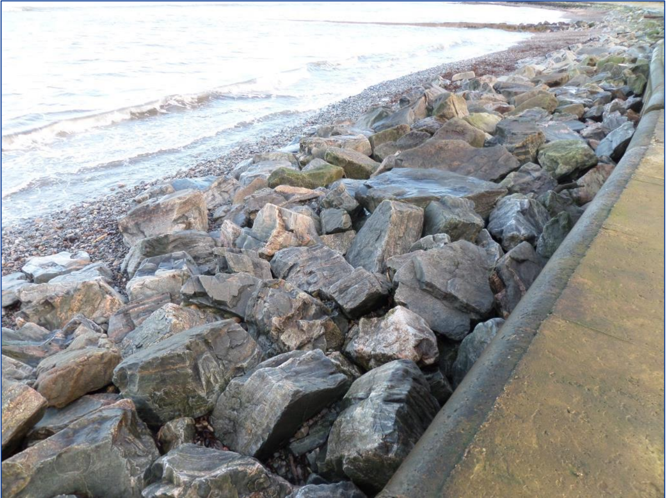
Figure 2-2: General view of rock armour in reasonable condition (2016).
