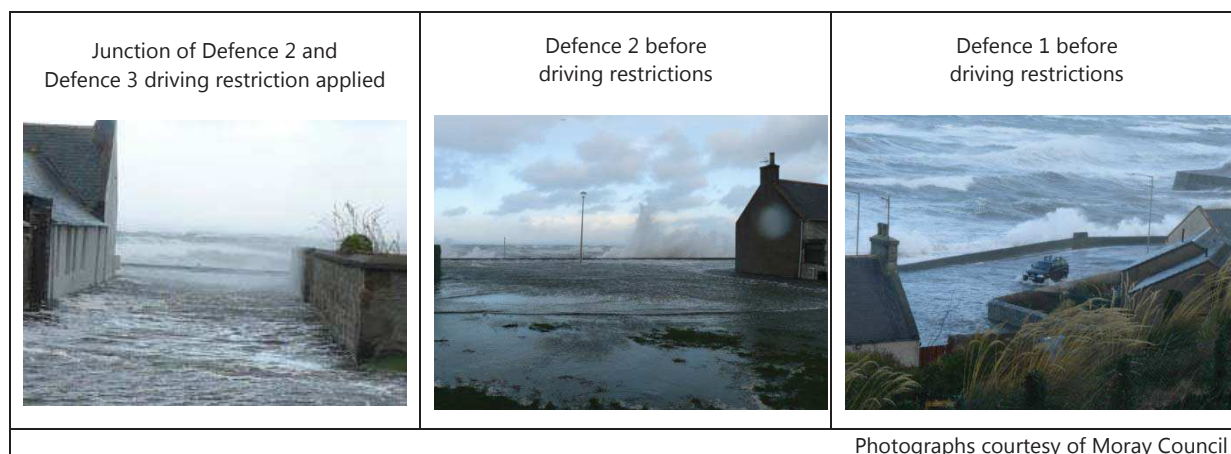
Figure 15. Photographic evidence of overtopping along the frontage for the 05/12/2013
