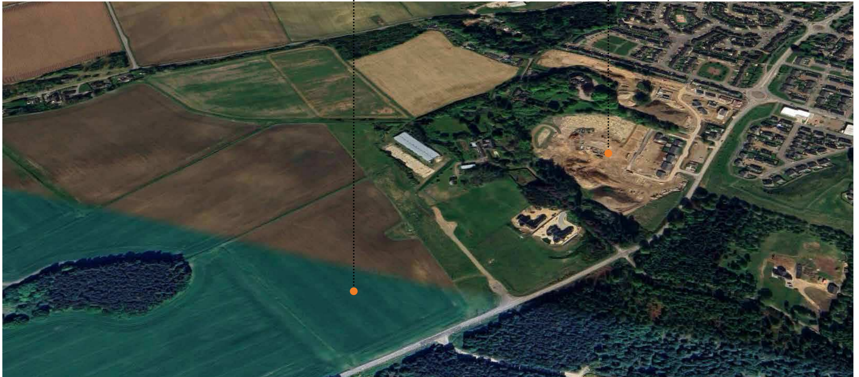
Aerial view of the Granttown Road site
