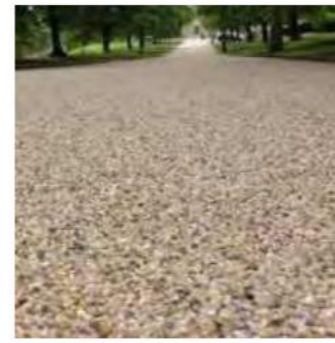
Surface aggregate overlay to give a natural looking surface suitable for heritage sites.
