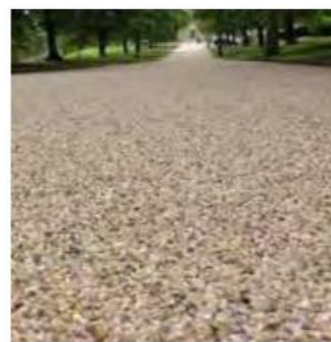
Surface aggregate overlay to give a natural looking surface suitable for heritage sites.
