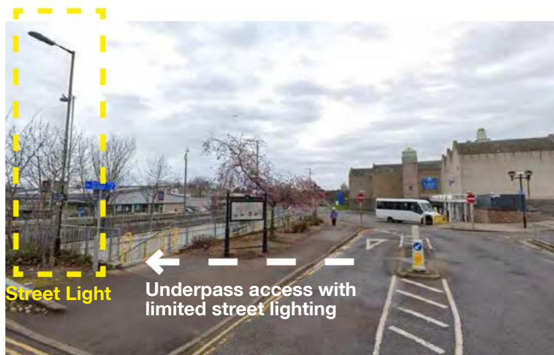
North Street - north entrance from the main street
