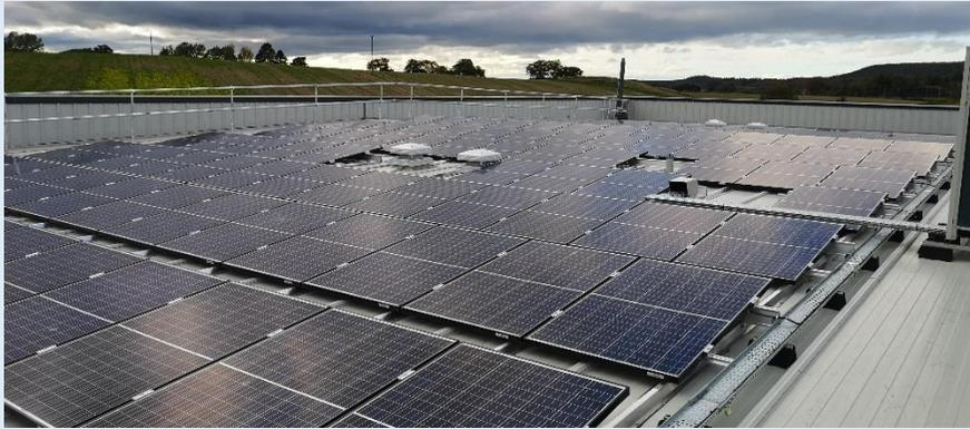
The council installed a 47kWp solar PV panel system at Elgin High School in October 2017. Since its commissioning, the system has generated over 177,491kWh of electricity and brought in over £5,000 in Feed-In-Tariff payments.
