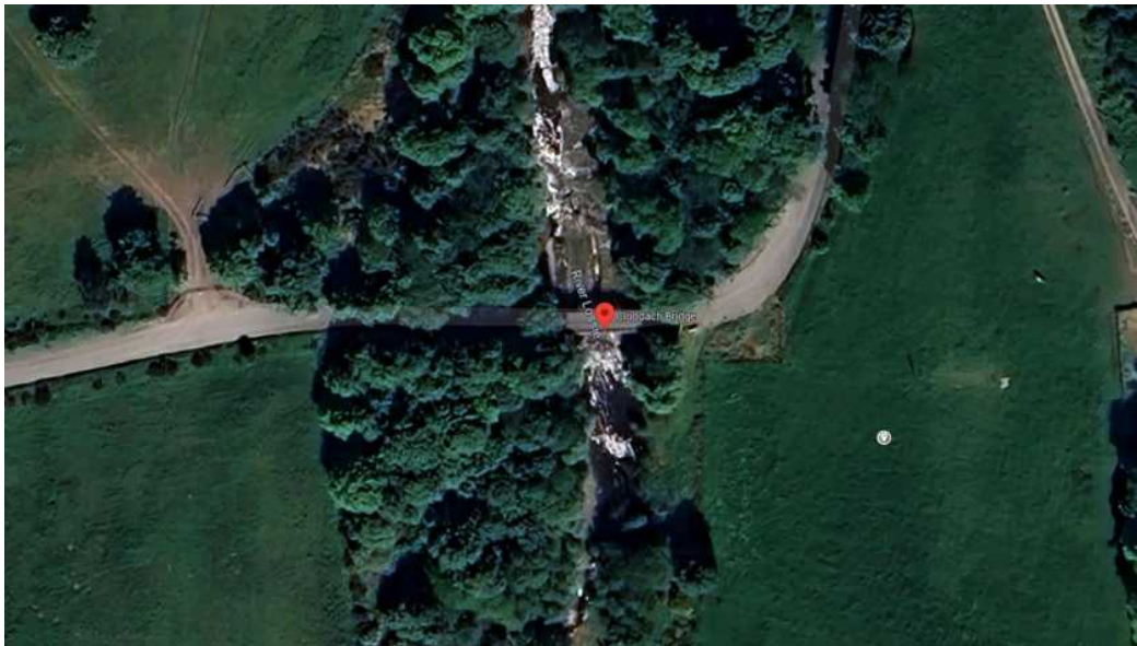
Figure 2: Bridge Aerial View
