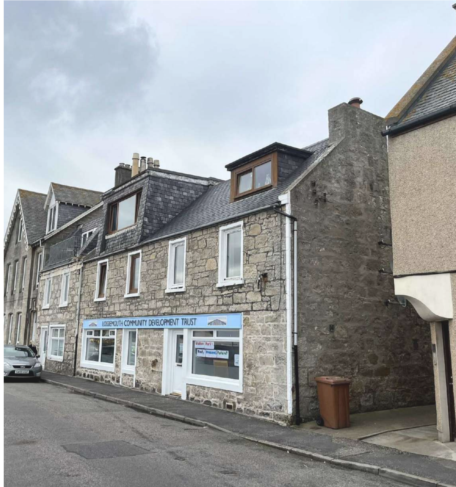
Image of Existing Street Front Elevation (1) Not to scale
