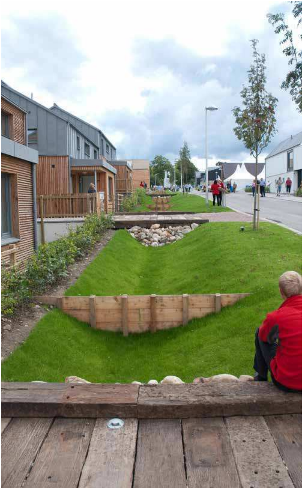
Swales integrated into residential layout to collect and treat surface water while also creating an engaging landscape feature.
