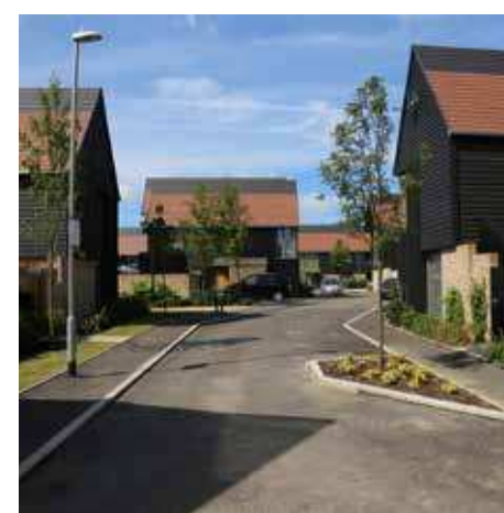
Throttle used to narrow the carriageway and reduce speed
