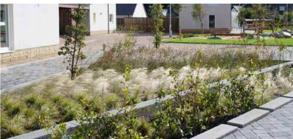
More structured and formal 'rain gardens' which gather and hold storm water during events and slowly release water back into the environment in a controlled rate. Bilbohall Masterplan
