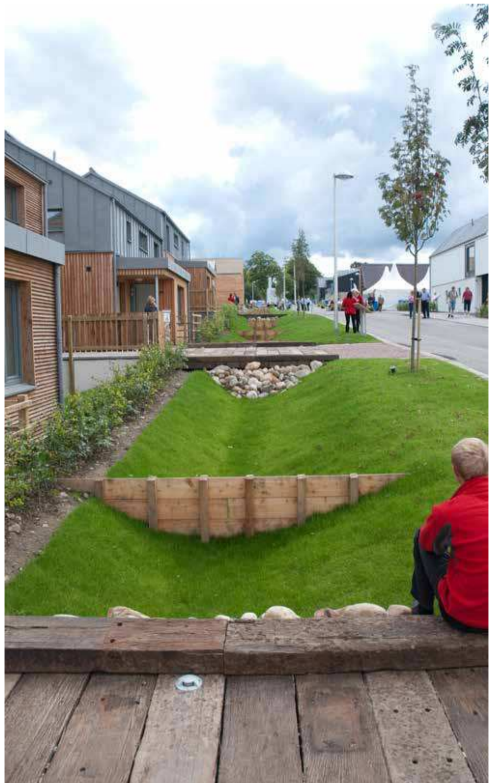
Swales integrated into residential layout to collect and treat surface water while also creating an engaging landscape feature.
