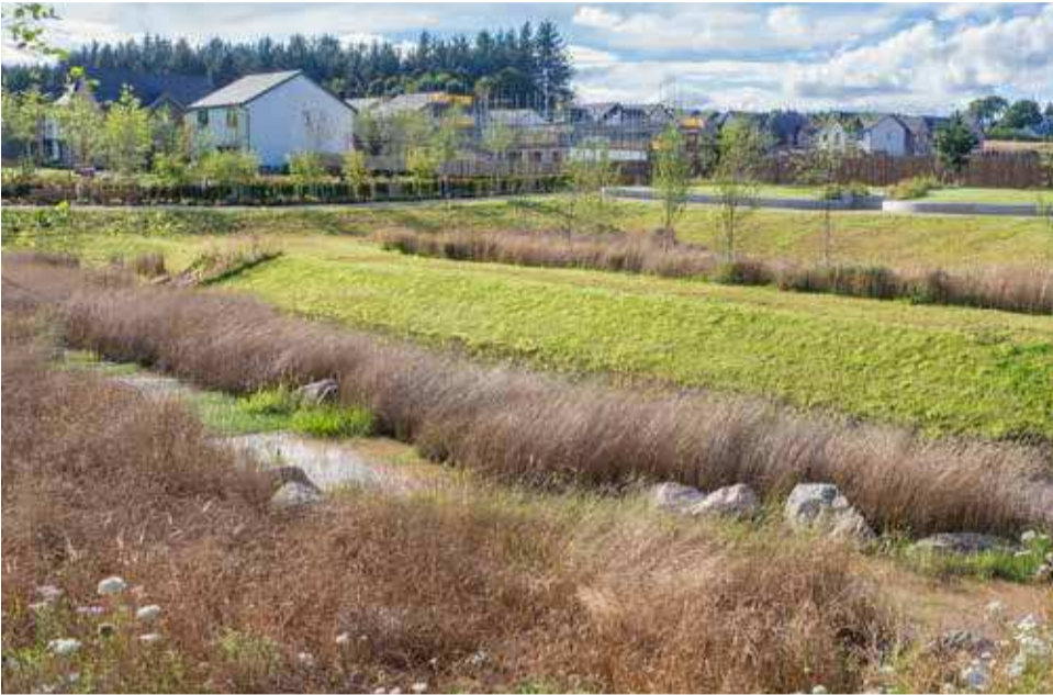
Interconnected SUDS basins with two levels of treatment, including wetland channels and areas and drier secondary basins.
