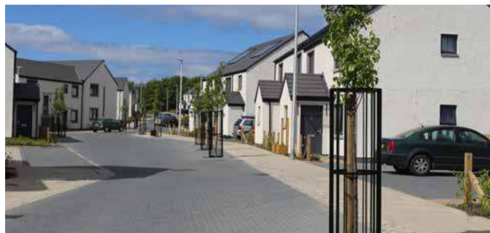
Vertical features and planting influencing the spatial feeling and therefore perception of speed for street users
