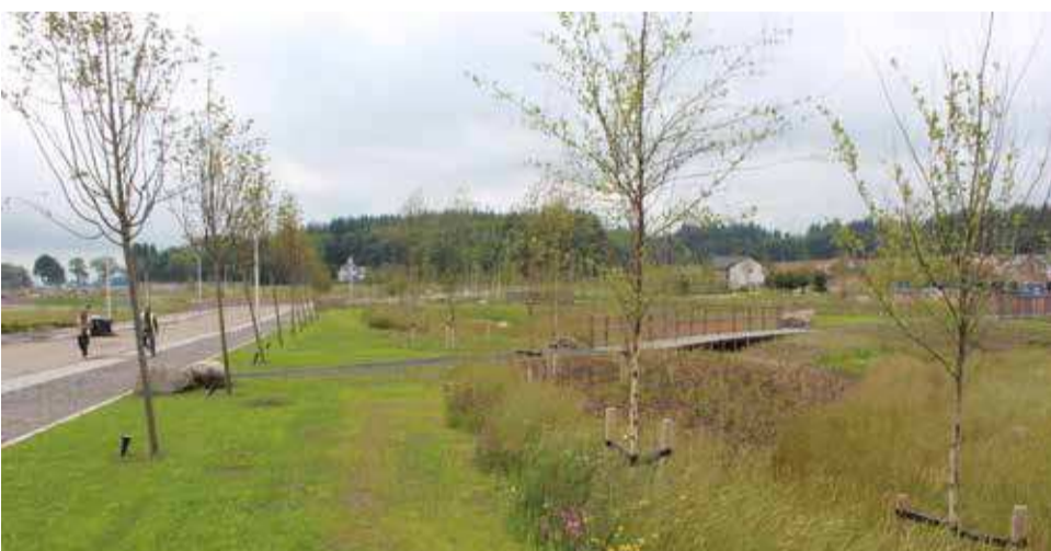
Water and SUDS systems adjacent to street network, providing open space with biodiversity benefits.
