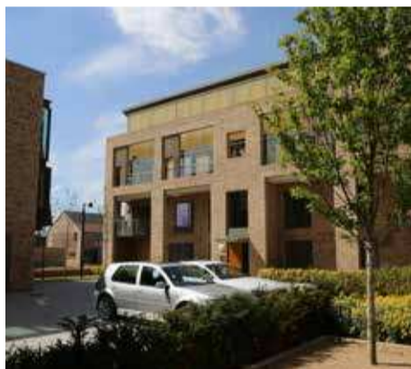
Parking courtyard overlooked with good integrated landscape structure and privacy.
