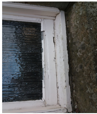
North Elevation Bathroom window, rotten cill ,window frame, sash boxes
