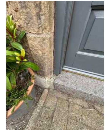
010 front door jamb/cill/step stone detail
