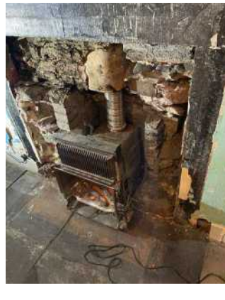
037 east living room original gas fire back boiler during removal 2021
